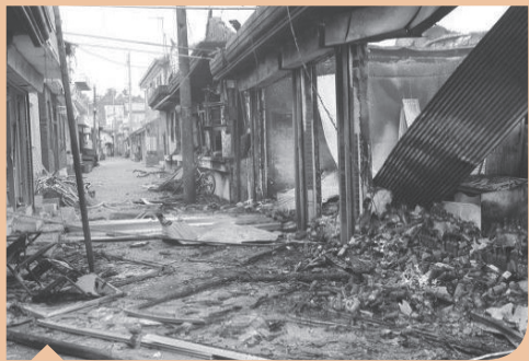
Private houses destroyed by North Korea's shelling of Yeonpyeong island
