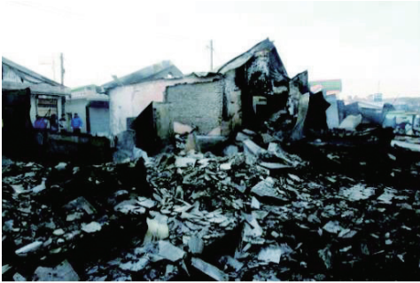
Houses damaged by North Korea's bombing of Yeonpyeong-do Island (November 23, 2010)
