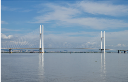
Amnok River Bridge (May 2020)
