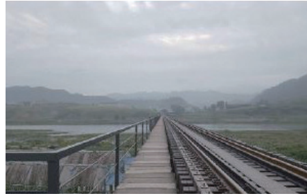
Railway between Jipian – Manpo (July 2017)
